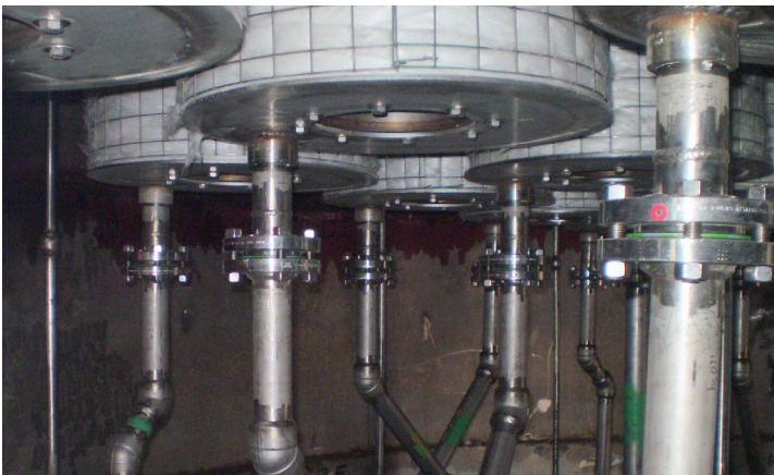
WITHOUT BRINK® AUTODRAIN™ seal legs, seal cups and complex drain piping are required, adding to the overall cost of operation.
