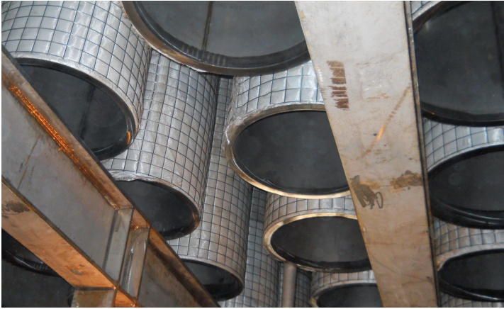
WITH BRINK® AUTODRAIN™ seal legs, seal cups and complex drain piping are not required for hanging fiber bed mist eliminators.
